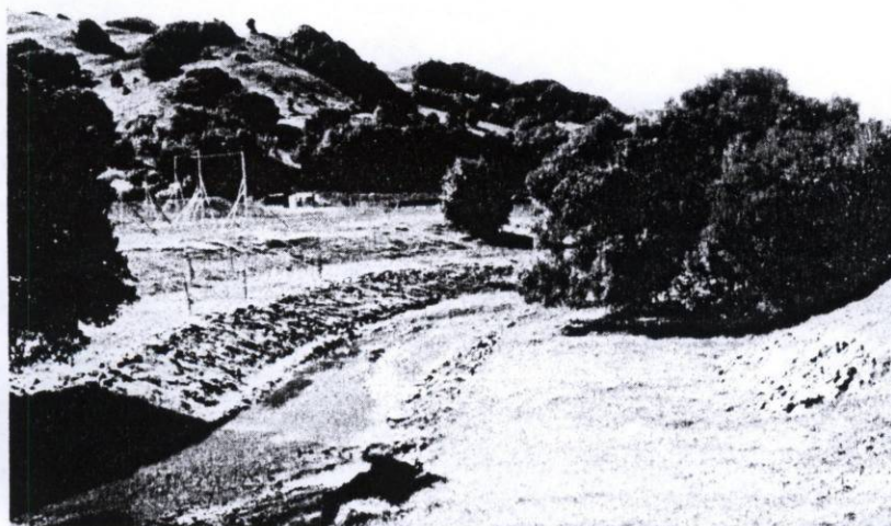
After: Grading to create two-stage channel
